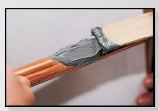
5. Cover area around pipe hole/crack.
