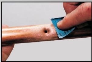
1. Prepare Surface around damaged area with sand paper or a file.
