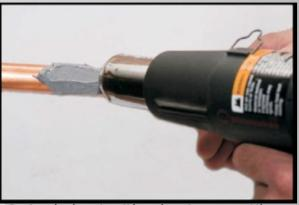
Apply heat with a heat gun until PIPESEAL cures and hardens within 1 minute.
